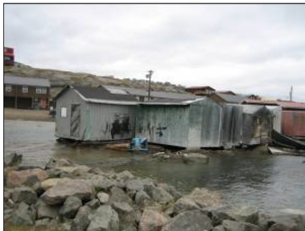
Flooding in Iqaluit, September, 2007
