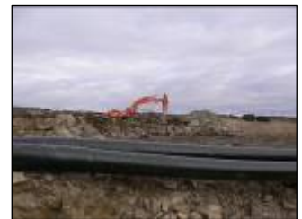
Backhoe installing underground piping.
